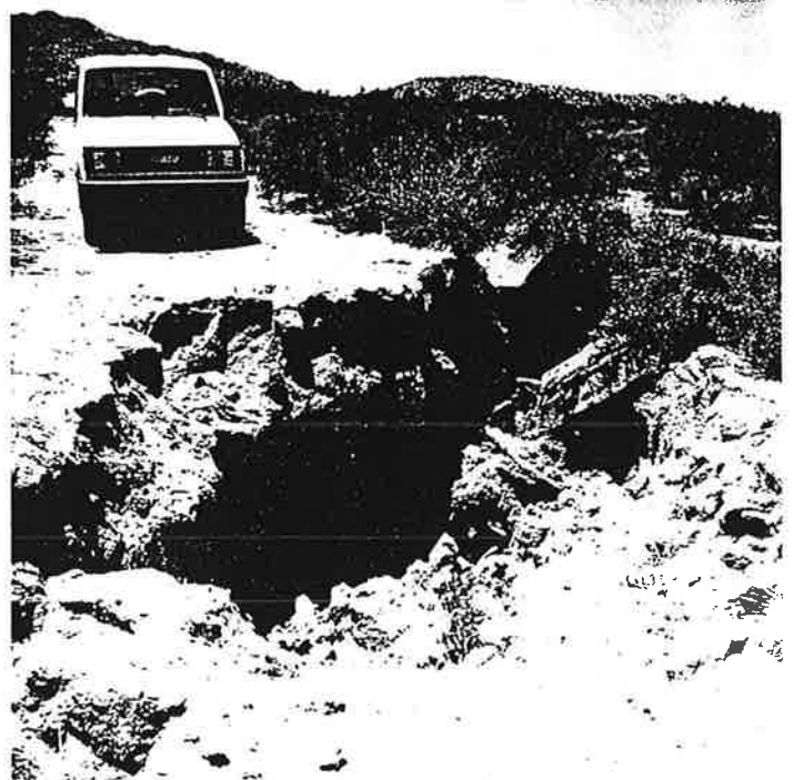
Figure 4. An earth fissure cut this road in Pinal County several miles east of Chandler Heights. Photograph by R. C. Harris.
